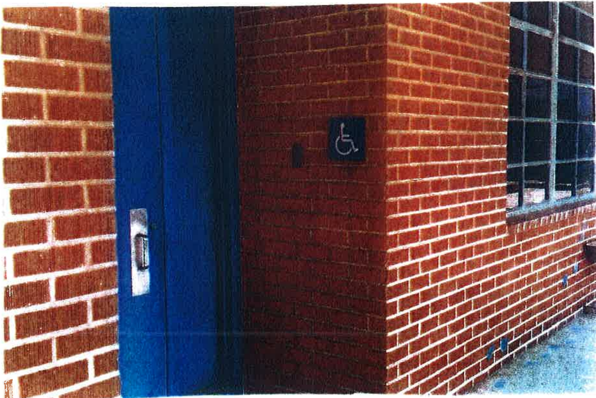
Photo #2: ADA accessible restroom at North School.
