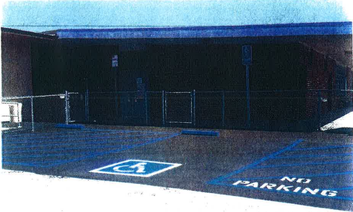
Photo #1: ADA accessible parking in the rear parking lot of North School. (There is also an ADA accessible parking space on the East side of the North School campus.)
